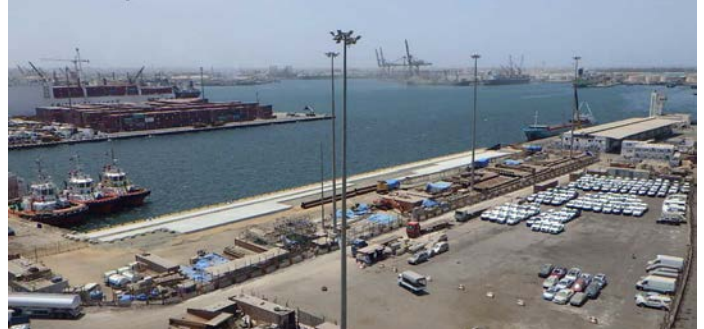
Fig. 6 Rehabilitation of Third wharf (After construction) in Senegal
