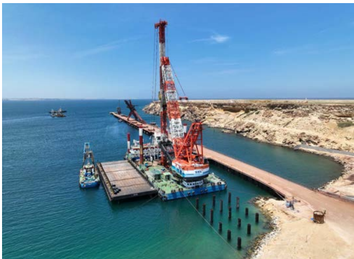
Fig. 2 Construction of Iron Ore Jetty Sacomar (Angola)
