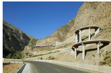
Fig. 1 Construction of N70 Project, Pakistan
