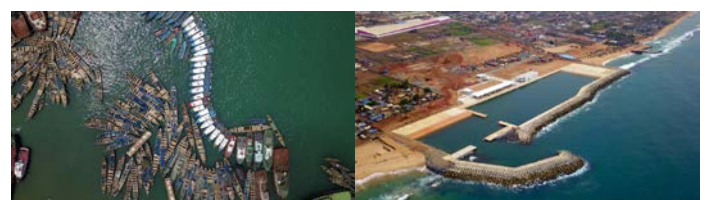
Fig. 4 Left (Old Fishing Port in Togo) Right (New Fishing Port after construction in Togo)
