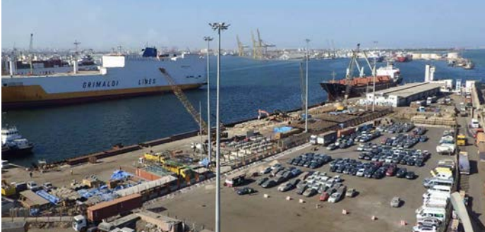
Fig. 5 Rehabilitation of Third wharf in Senegal (During construction)
