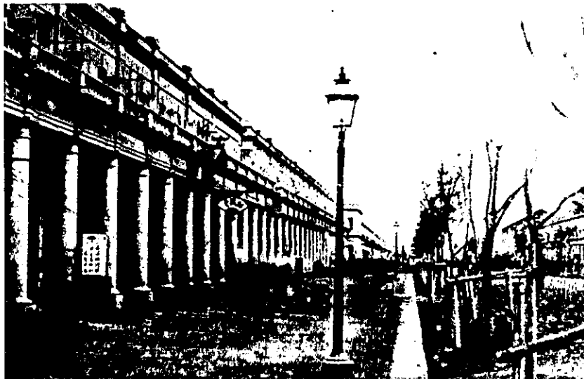
Figure 2 Ginza street (completed in 1877)
